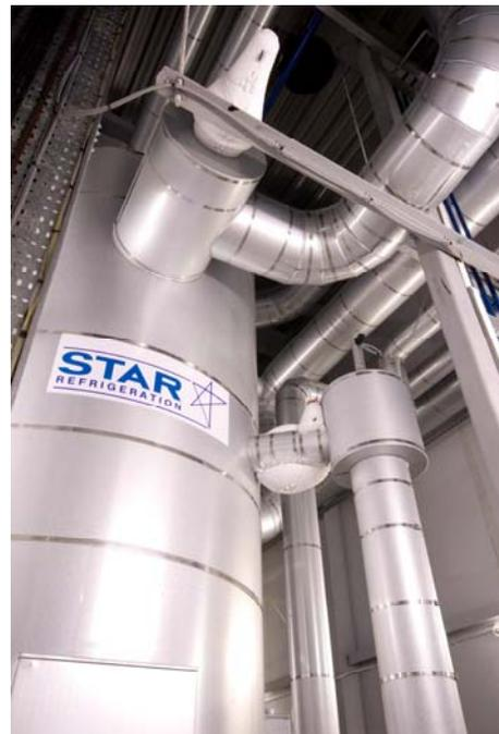
**Chill store vertical surge drums, designed to meet space constraints in the site's purpose built Energy Centre.**
