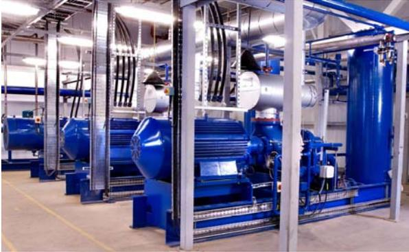
Star built low stage screw compressors, including variable speed drive on the far end compressor.
