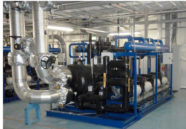
Inside the plant room - Star's high efficiency chiller package for data centre cooling
