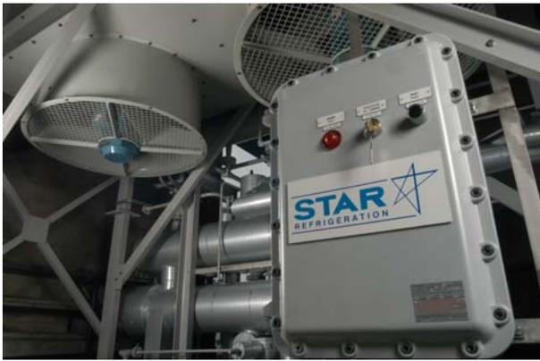
View showing skid mounted control panel
