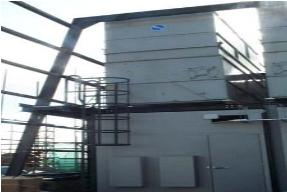
The chiller housings and condensers during installation.
