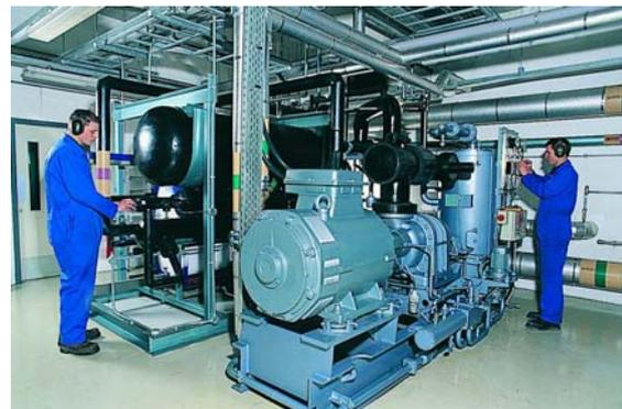
The total ammonia content is just over one tonne, with charges for phase 1, 2 and 3 of 450, 250 and 350kg respectively. The modular LPR configuration allows a much lower charge than the equivalent pumped central plant system and also
