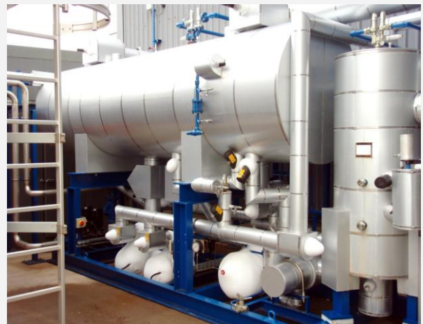
Star handled the removal of the existing R22 plant
