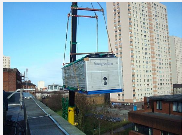
A crane lifting one of Star's Indigochillers into position on the roof of the Curran Building at the University of Strathclyde.
