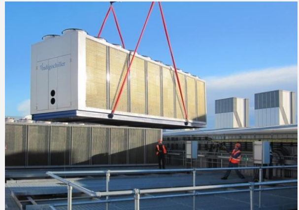
One of Star's Indigochillers being lowered onto the roof of the new Sky Studios building
