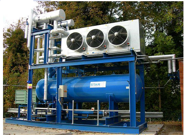
Star Refrigeration's thermodynamic dual-purpose gas recycling system, developed for Alstom
