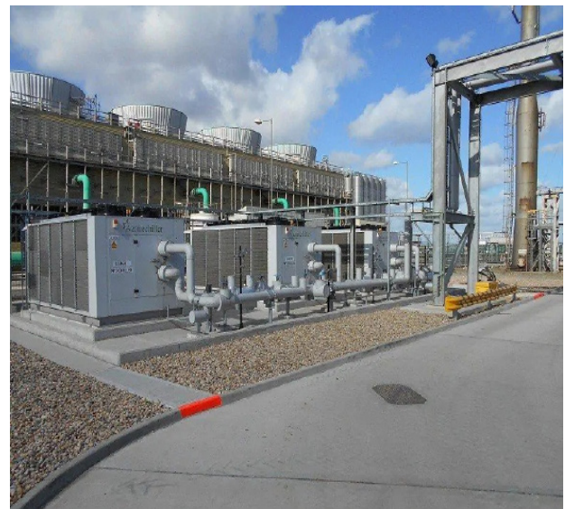
-18oC Air-Cooled Fluid Chillers in Petrochemical Application
