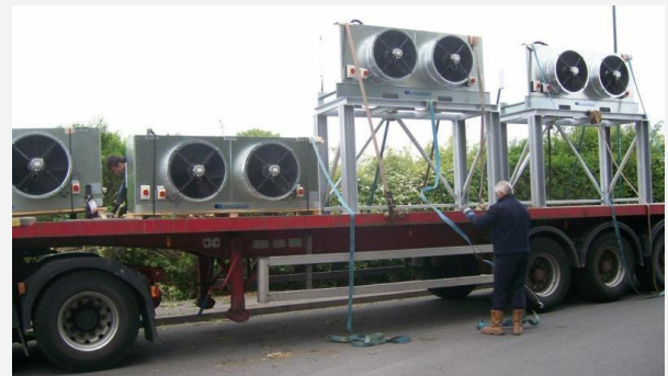
Pre-assembled air cooled units being delivered to site at MKG
