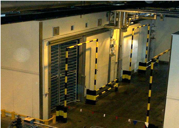
Two of the ten blast freezers at Lerwick, installed to increase capacity
