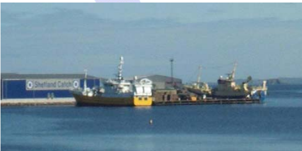
Trawlers berthing alongside the new Shetland Catch factory on the quayside
