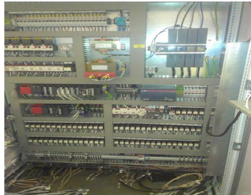
Each of the 4 Control Panels incorporated 1 off Mitsubishi Q Series PLC Control & Monitoring System – "Telstar PLC"
