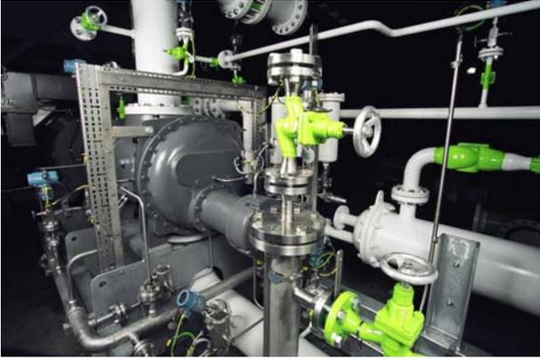
To provide a degree of in-built equipment reliability, the compressor package was designed with dual oil pumps and dual oil filters thereby ensuring that filters could be changed while the compressor was operating.
