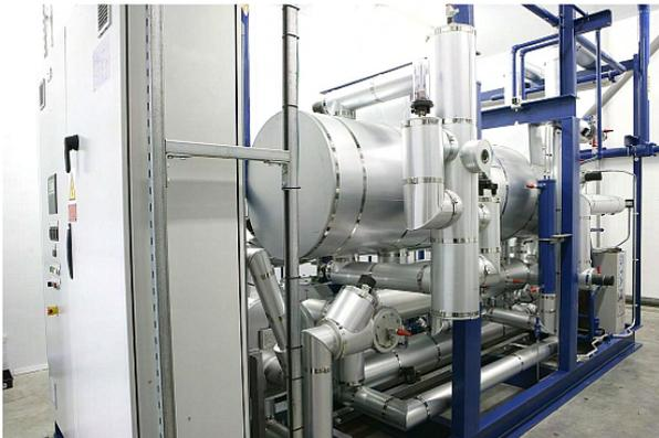
Part of Star's state-of-the-art refrigeration plant, which provides cooling for three cold stores at Chan Brothers.
