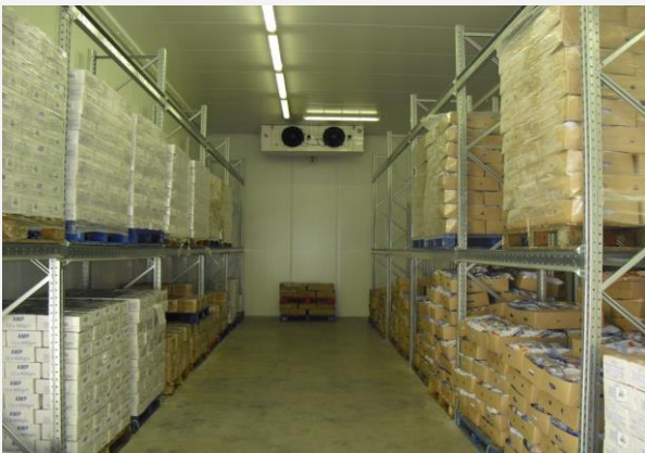
A Guntner evaporator within the cold store chamber at Anglian Meats depot
