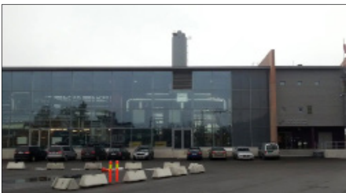
Star's Neatpump plantroom in Drammen
