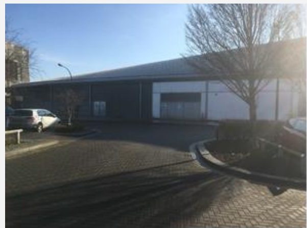
External area for new ammonia chillers
