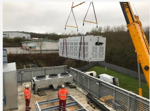
The Blakemans project was completed following a carefully phased 15-week installation programme which required the temporary relocation of the existing coldstore condensers to make space for the Azanefreezer. Star's expert engineering team carried out decommissioning and disposal of all existing equipment, whilst maintaining temperature continuity and ensuring 24/7 operation in both cold
