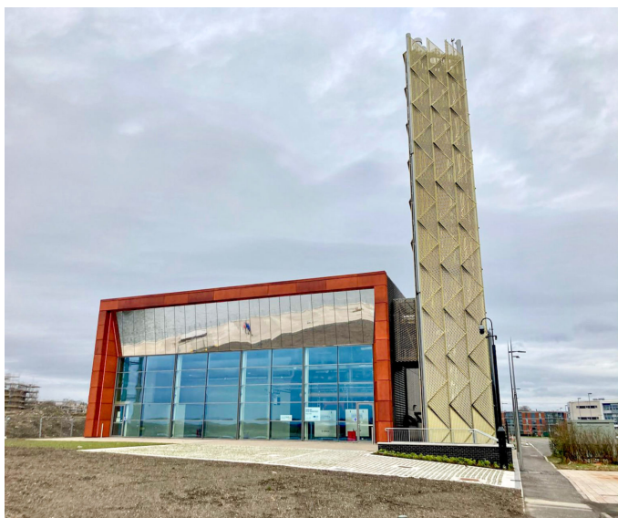
Scotland's first large-scale water source heat pump
