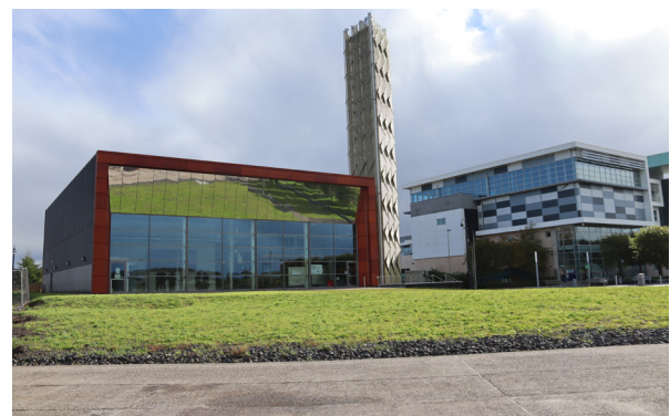
Clydebank Energy Centre where Star's water source heat pumps for district heating are housed
