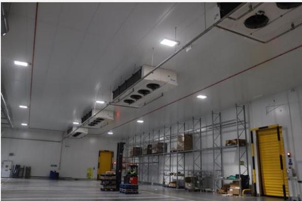
The refrigeration system is fitted with a heat recovery system designed to repurpose waste heat to the underfloor heating mat and facilitate warm glycol defrost on the air coolers. The heater mat installation uses stainless steel pipework headers and a Medium-Density Polyethylene (MDPE) underfloor pipe. Each pipe has been equipped with individual valves and flow indicators to allow for precision control and monitoring.
