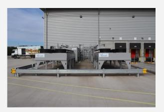
Star's CO<sub>2</sub> based refrigeration system is located externally, adjacent to the building and serves the main freezer chamber and accompanying chill stores at Bidfood's Glasgow facility. The site also
