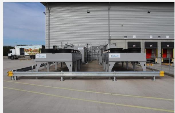
Star's CO<sub>2</sub> based refrigeration system is located externally, adjacent to the building and serves the main freezer chamber and accompanying chill stores at Bidfood's Glasgow facility. The site also
